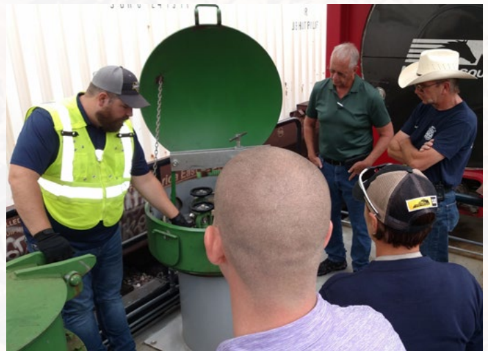
Brian Shanks (Norfolk Southern) explains the chlorine valves and the Chlorine Institute Emergency C kit that is in place.
