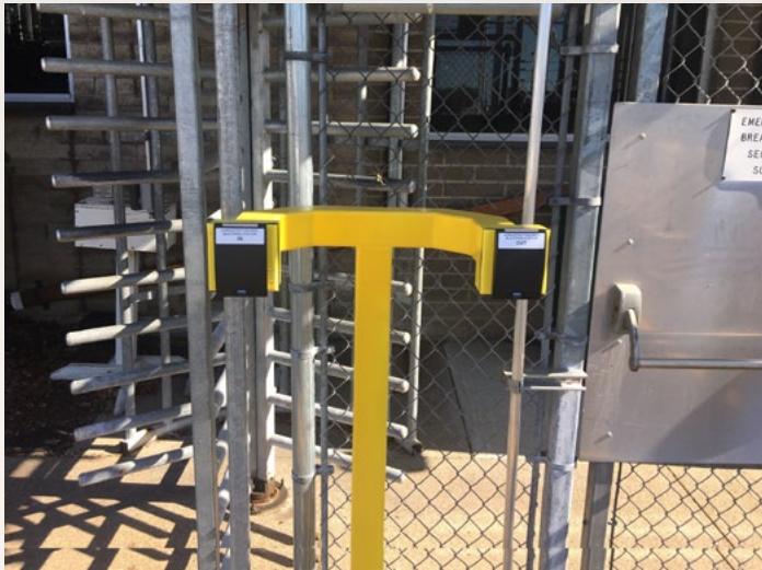
Figure 1: Many facilities have a computer badging system that employees use to get inside the fenceline and any secure areas within the facility. These same systems can be used to obtain employee accountability during an emergency. In this case, during an evacuation, the employee badges in at the muster station and badges out if they leave the muster station.
