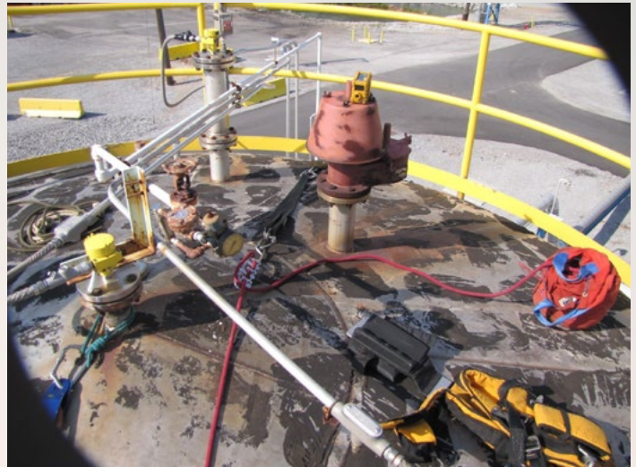
Figure 2: Always consider the potential hazardous materials aspects of all incidents inside the fenceline. The incident you are handling may not be associated with this tank. However, operating on or near the tank could pose a hazard due to vapors coming from flanges, valves, and/or vents.
